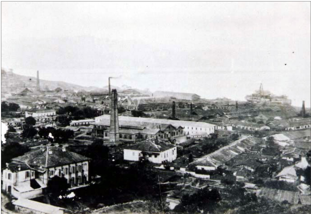
FIGURE 9.25 Fuzhou Arsenal. The Fuzhou Arsenal in Mawei was built as part of China's Self-Strengthening Movement. This photograph was taken in about 1880. (credit: "Foochow arsenal in Mawei" by Unknown/Wikimedia Commons, Public Domain)
