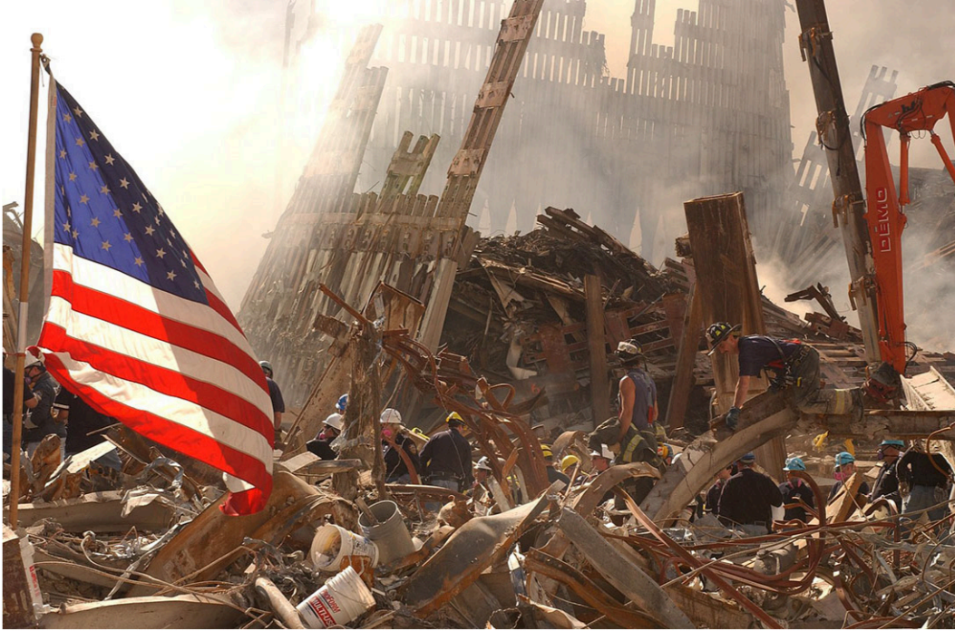
FIGURE 15.24 September 11, 2001. Less than two hours after hijackers flew two jetliners into the World Trade Center in New York, both its towers crumbled to the ground in a pile of rubble. Those still inside were all killed. (credit: “New York, NY, September 19, 2001 -- Rescue workers climb over and dig through piles of rubble from the destroyed World Trade Center as the American flag billows over the debris” by Andrea Booher/Wikimedia Commons, Public Domain)
