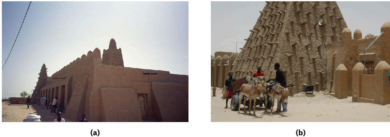
FIGURE 15.10 The Djinguereber Mosque. (a) (b) Fourteenth-century Timbuktu was a great center of learning specializing in Islamic law, philosophy, and science. These photos show two views of the famous Djinguereber Mosque, built there in 1327. (credit a: modification of work “Djinguereber Mosque, Timbuktu” by “upvernoz”/Flickr, CC BY 2.0; credit b: modification of work “Timbuktu Mud Mosque, Mali, W. Africa” by Emilio Labrador/Flickr, CC BY 2.0)
