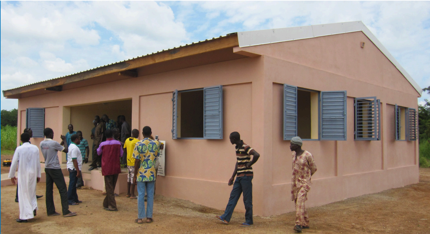
Figure 17.1 The US Army Corp of Engineers opened this community health clinic in the country of Benin in West Africa in 2013. The clinic has waiting, consultation, observation and treatment rooms, and a drug store. (credit: “Pehunco Health Clinic opens” by US Army Corps of Engineers/Wale Adalakun/flickr, Public Domain)
